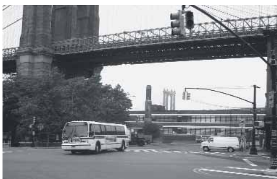
EXISTING CONDITIONS Old Fulton Street looking north to the Purchase Building
