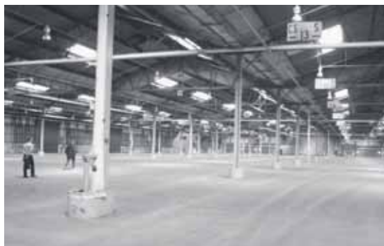
EXISTING CONDITIONS Pier 6
