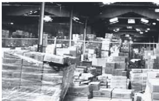
EXISTING CONDITIONS Pier 5 shed
