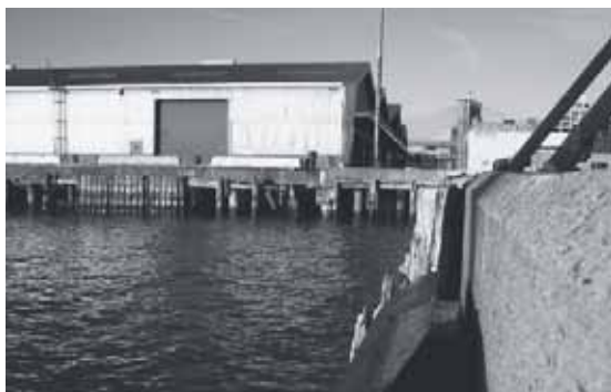
EXISTING CONDITIONS Bulkhead between Piers 2 and 3
