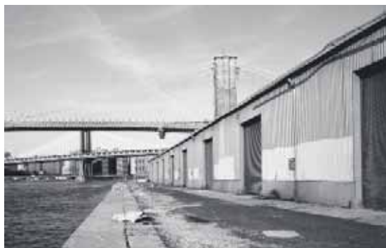
EXISTING CONDITIONS Pier 1 looking to the Brooklyn Bridge
