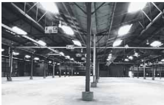
EXISTING CONDITIONS Pier 2 shed
