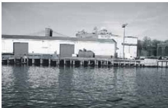
EXISTING CONDITIONS Pier 2 looking North to Pier 1
