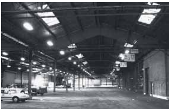
EXISTING CONDITIONS Pier 2 shed
